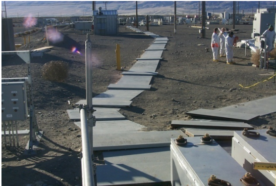
HIHTL in shallow trench covered by steel plate
