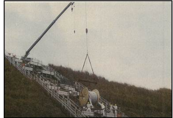
HIHTLs being installed at Fukushima nuclear plant
