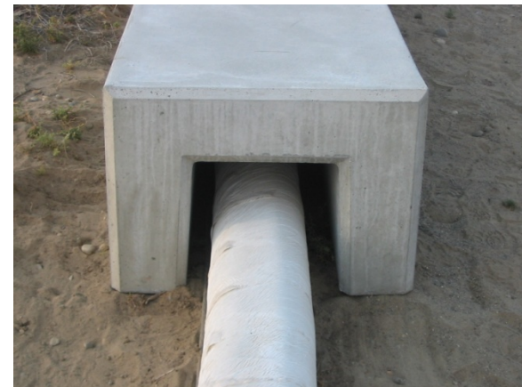
HIHTLs at grade level, shielded by concrete hose "barns"
